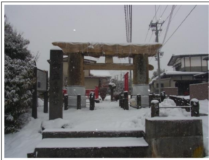
Fig. 1: Stone shrine gate with winter cover in Motoki, Yamagata city.
