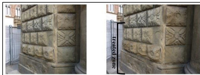
Fig. 7: The sandstone before (left) and 30' after the \text{TiO}_2 application (right).
