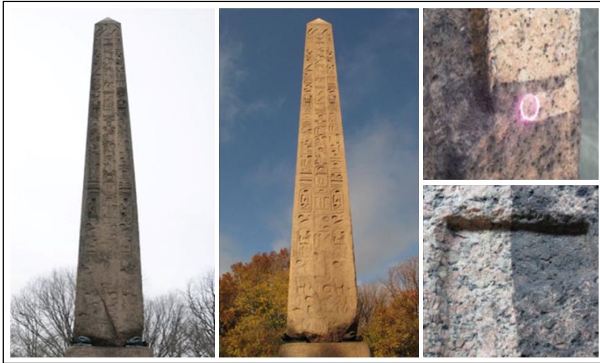
Fig. 8: Overall and detailed results of laser cleaning the obelisk.
