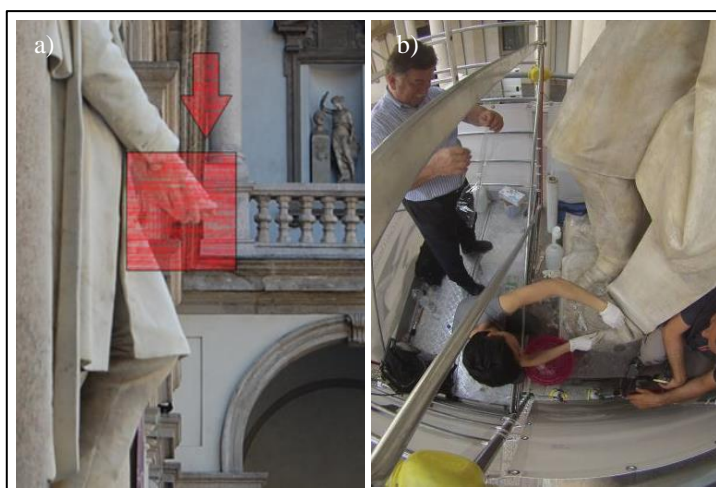
Fig. 7: a) Scheme of the consolidation system adopted (dip coating); b) Dr. Annalisa Balloi during the application of sulfate-reducing bacteria through a gelatinous medium on the areas that were altered and covered by sulfates.
