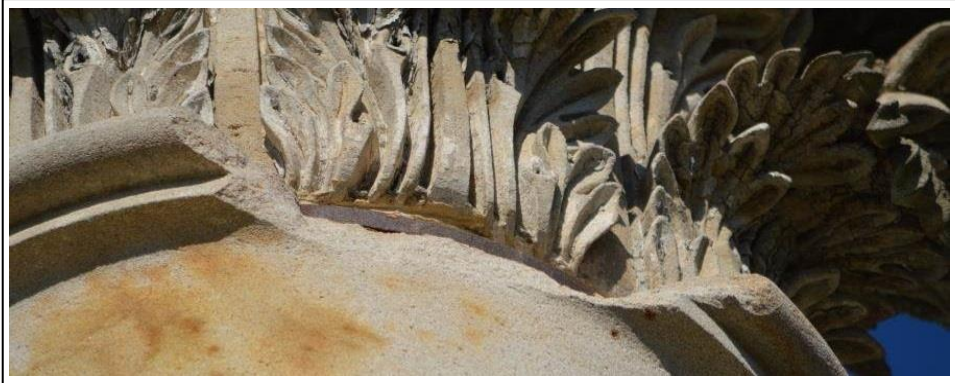
Fig. 7: Detail of stone loss from L13's astragal, revealing its iron ring directly below the bottom edge of the capital.
