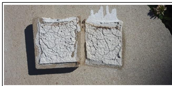
Fig. 6: Grout applied to two sandstone surfaces remained secure for 45 days at which point it was separated. The bond was adequate but lower than ideal. The inner surface showed a network of cracks that no doubt contributed to this. The shrinkage is considered to be the result of the stone sucking liquid from the grout too quickly, emphasizing the need for adequate pre-wetting of the inner surfaces.
