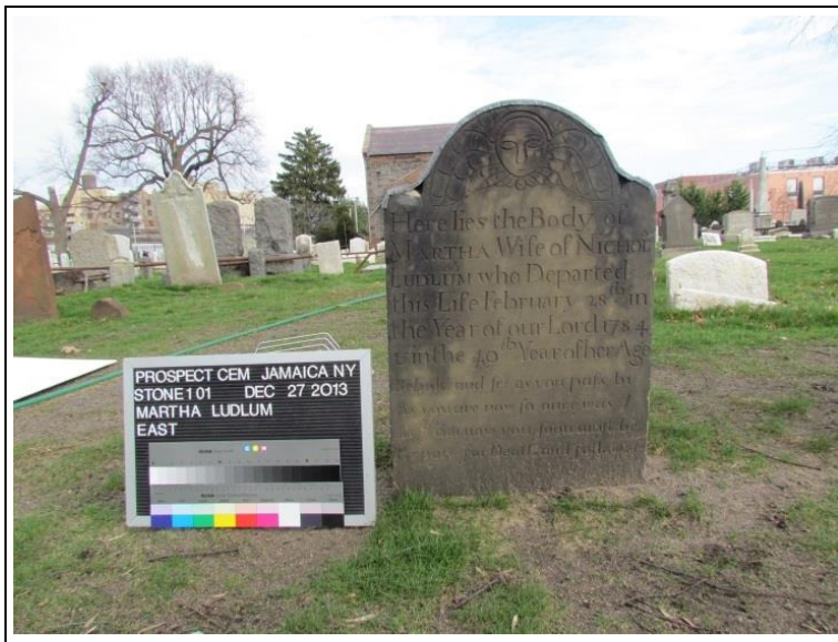
Fig. 4: Lead cap over delaminating sandstone marker.
