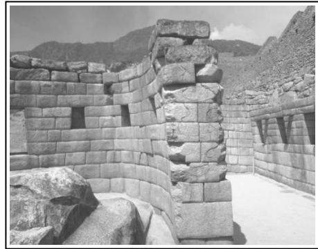
Fig. 6: Missing parts of edge stones.
