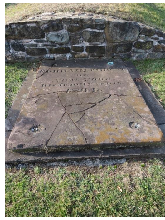
Fig. 1: Vault Slab with Pinning Repair 10 years later.
