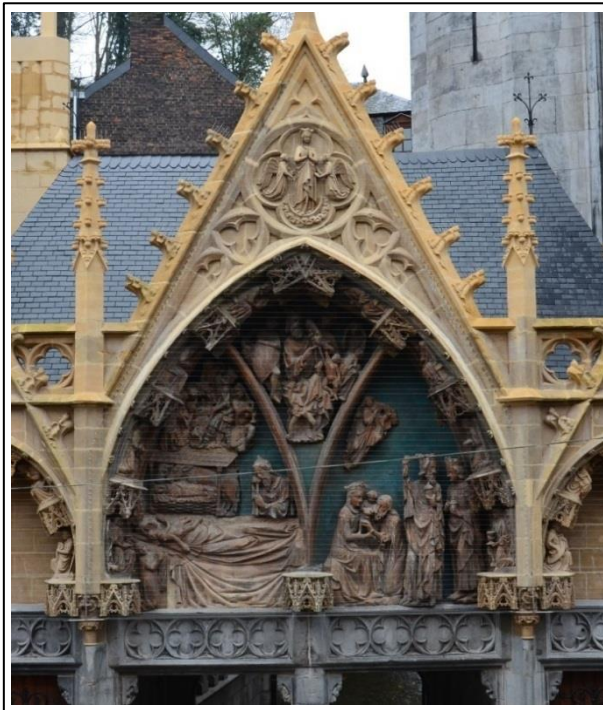
Fig. 8: Portal after maintenance treatment in 2014.
