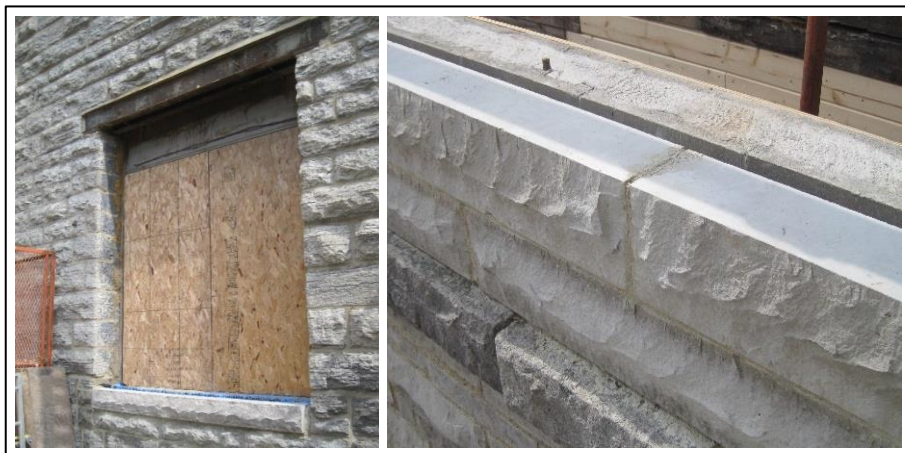
Fig. 4: Representative examples Lannon stone used as a substitute for Platteville stone. Image on the left is a replacement sill and image on the right is a reconstruction of a parapet.
