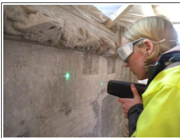
Fig. 3: Desoiling using Nd:Yag Conservation Laser System.
