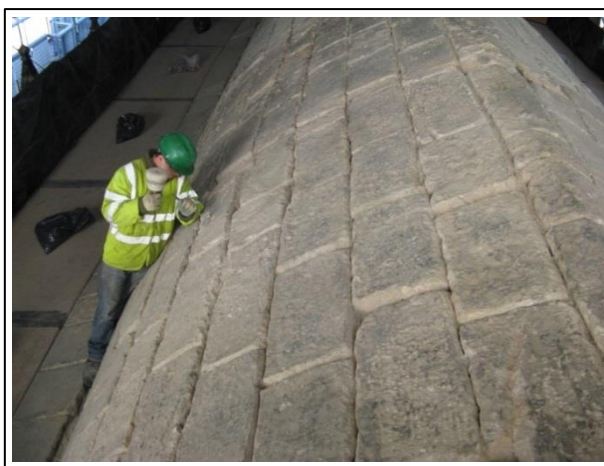
Fig. 1: Raking out vault joints.
