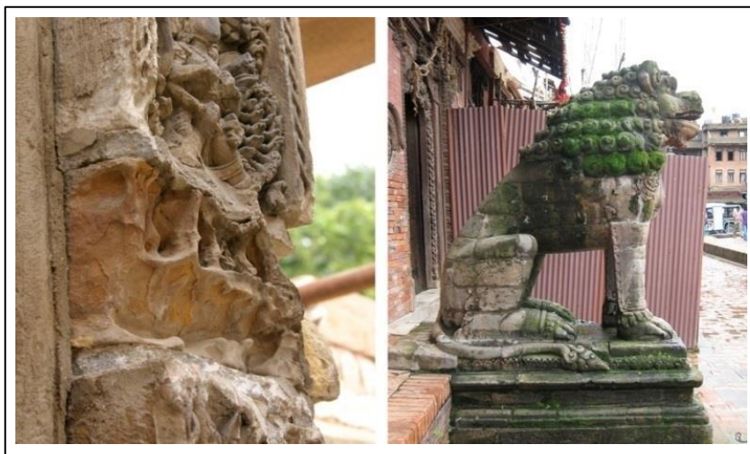
Fig. 1: Decay patterns and typical construction of monuments made of the siliceous sandstone.
