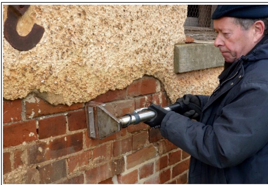
Fig. 1: Captive-head washing system being used by Walter Heim to remove dust and dirt from brickwork prior to render repairs at Brickendon, Longford, Tasmania.
