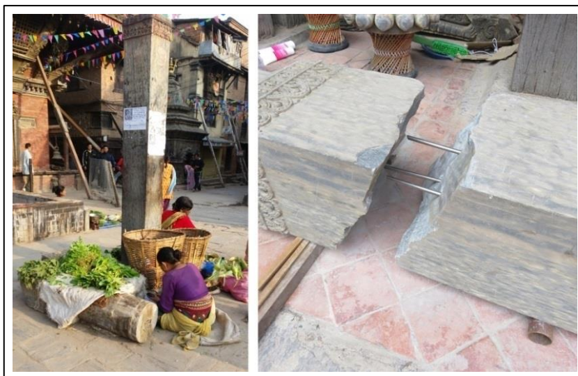
Fig. 3: Partly collapsed pillar used as market stand (left), gluing of broken parts (right).
