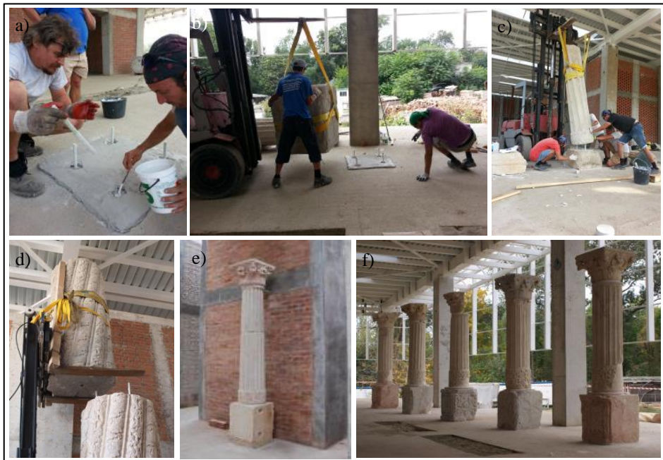
Fig. 5: Installation of the columns: a and b) Bottom pin structure, c to e) Assembly of the decorated stone block to columns in the Royal House; f) Columns of the veranda.
