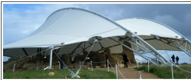
Fig. 1: Shelter over the megalithic temples at Hagar Qim, Malta.
