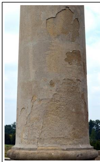
Fig. 6: Same location as the previous in 2013, showing an estimated 10-15% additional contour losses after 25 years.
