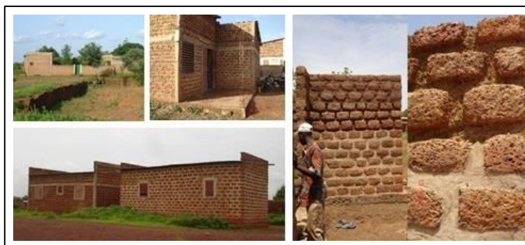
Fig. 2: Typical houses in LDS, either load bearing masonry or with frame concrete.
