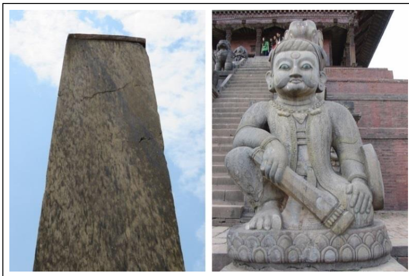
Fig. 2: Decay patterns and typical construction of monuments made of the metamorphic stone.
